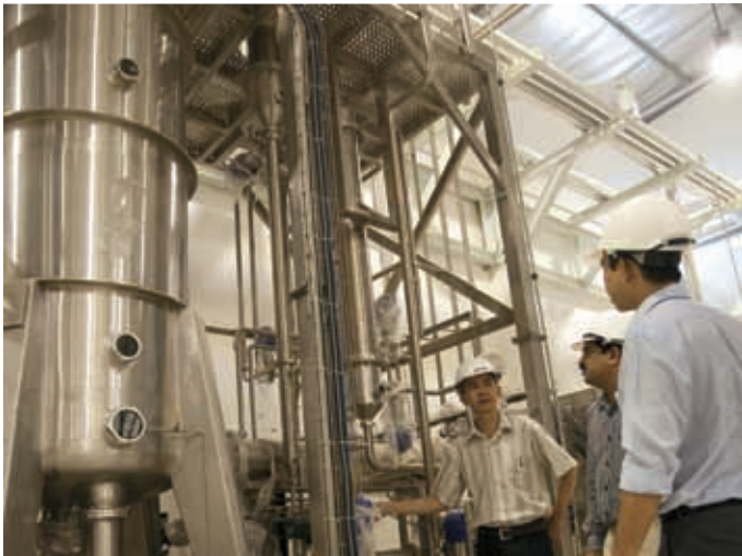
Soluble coffee manufacturing, Ho Chi Minh, Vietnam: The facility is expected to commence production from November 2009 and contribute to margin growth in FY2010.
