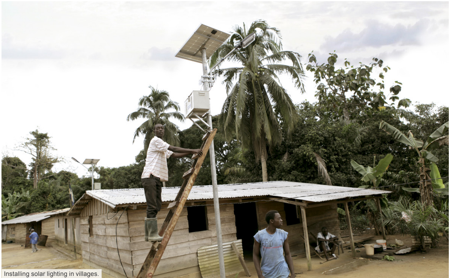
Installing solar lighting in villages.
